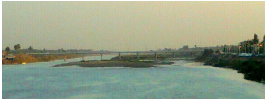
Figure 2: Al- Hindiya Second Bridge
